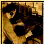
In this electric oven the "climate" is laked out of SCOTT transformers. After every lot of moisture is laked out, the parts are tested so that they will always deliver perfect service in any climate from that of the Arctic to the humid heat of the Tropics.
